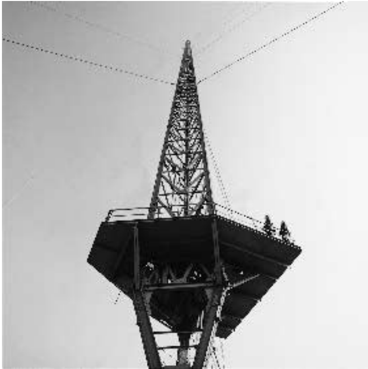
Figure 6.5. One of the two 250-metre masts supporting the MSF transmitting aerial near Rugby. MSF transmits continuous time signals on 60 kilohertz which are widely used to control radio clocks and other equipment.
