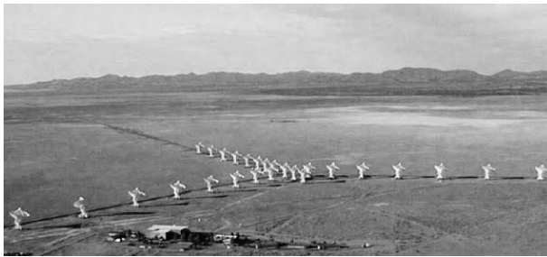
Figure 2. The Very Large Array (VLA) on the plains of St Augustine in New Mexico, operated by the National Radio Astronomy Observatory of the USA, contains 27 25 m diameter telescopes.
