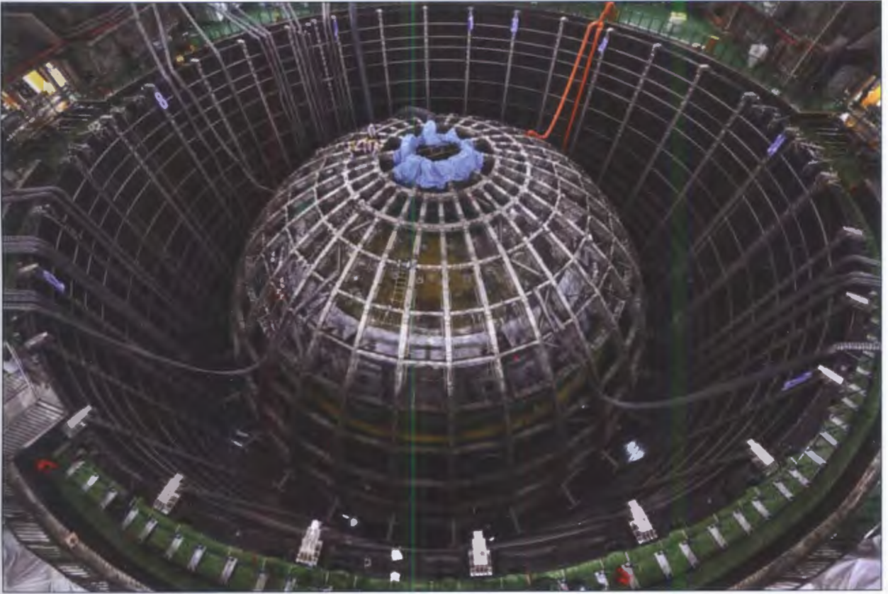
Fig. 17. Current status of the JUNO detector assembly
