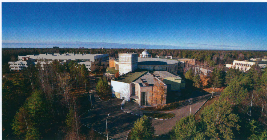
The building of the Synchrotron – the Nuclotron
