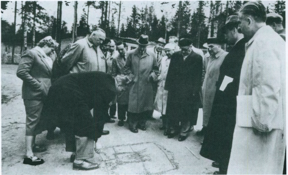
1956. Members of the JINR Scientific Council at the construction site of the new building for the Laboratory of Theoretical Physics
