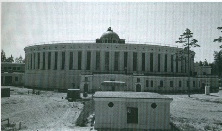
The main building of the Synchrophasotron
