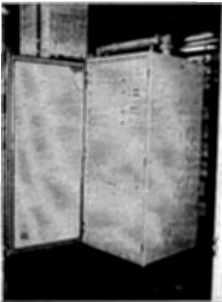
Fig.1: HF generator Georgit-2. 25kW, 38MHz.
