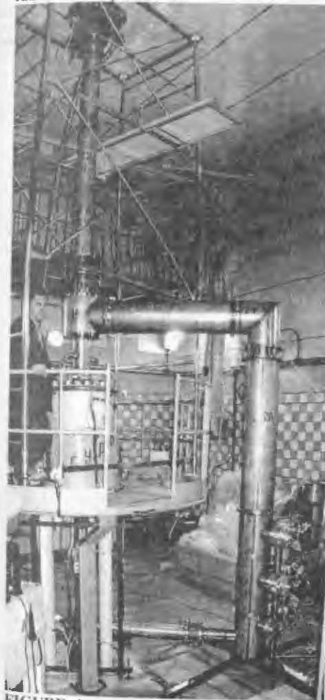
FIGURE 4. The installation of the set-up at the reactor
