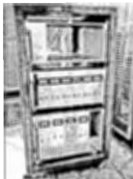
Fig. 3. Schematic of the distributed automatic stabilization sub-system for magnetic lenses (left) and photo of the rack with power supplies inside the accelerator hall (right)
