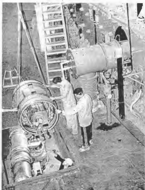
Figure 1. Transportation of the Lambertson magnet section in the tunnel
