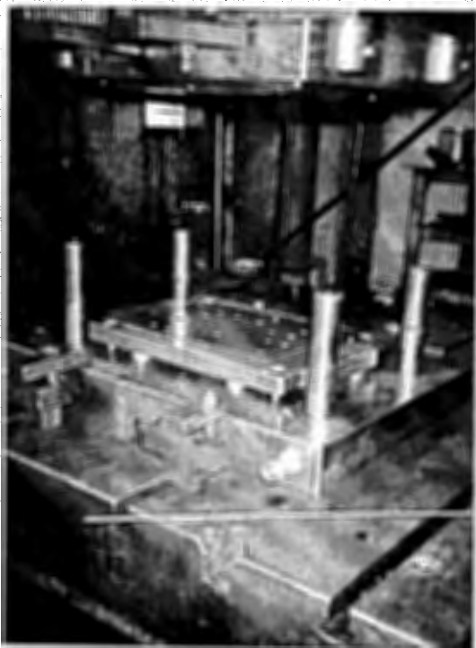
Fig's 6.7.- (photo)-Cutting die for spacer # 12 inserted into 500 t press (Belusa, Slovakia, December' 97).
