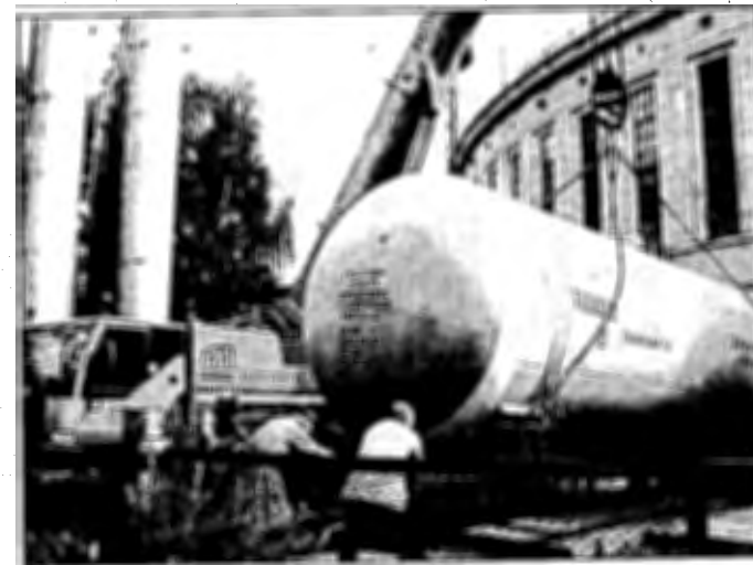
Fig. 21. The new liquid nitrogen storage vessel integrated into the Nuclotron cryogenic system.
